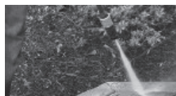
WASH FACADE USING NYLON BRUSH
