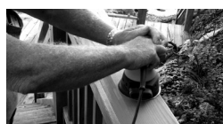
IF NECESSARY, FINISH SANDING
